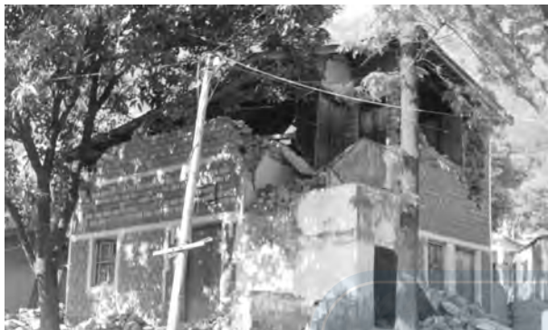
Figure 7.1 : A Damaged Building Due to an Earthquake
